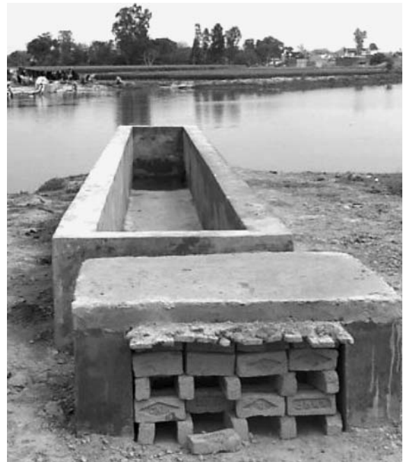
Fig. 3 A prototype of horizontal flow constructed wetland
